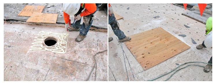
Repairs to openings in the concrete deck were easily accomplished with spray urethane foam and a plywood cover board to seal the opening. Air infiltration was eliminated with very little effort.
