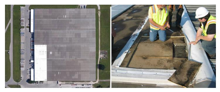
KOHLER FACILITY BEFORE Condensation from the building was collecting under the membrane, soaking the insulation and causing a great deal of problems inside the facility.
