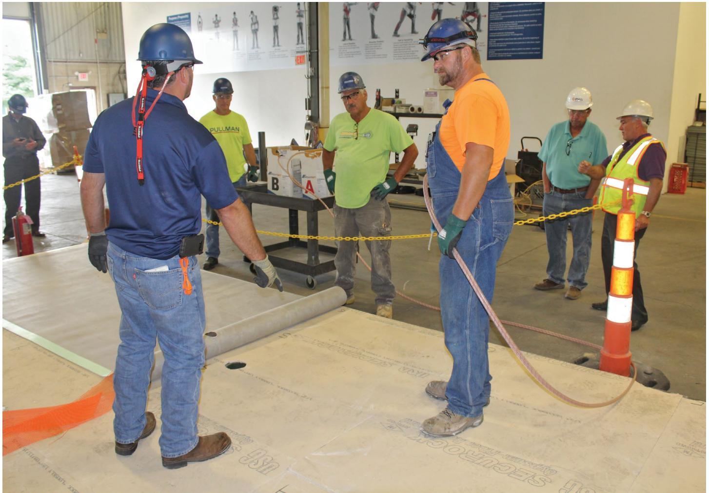
Under traditional circumstances, there would have been no way to anticipate installation needs unless actually on site. However, the low-profile design and simplified application of V2T meant that a life-sized roof mock-up could be created and rehearsed off site - and even demonstrated to the end client.
