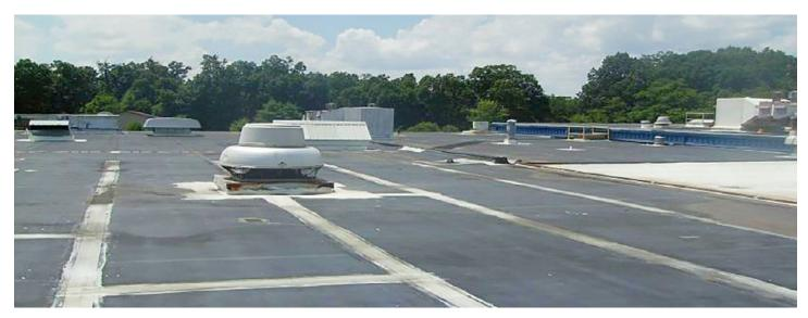
The roof was a metal deck with a gravel surface built-up (BUR) and a recovery roof with insulation board and 45 mil EPDM. The EPDM roof was so saturated that you could see footprints when walking over the roof. Acrylife surveyed the roof, took core samples, asbestos samples and recommended removal of equipment that was obsolete. After a complete investigation, Acrylife recommended that the roof be removed and a new roof be installed using Versico 60 mil PVC and the V2T Vent Technology.
