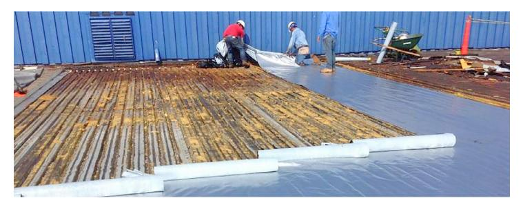
Because this was a complete tear off to the metal deck, Acrylife recommended using Carlisle's new VapAir vapor barrier over the deck. This is a new reinforced peel and stick butyl backed sheet that directly adheres to the deck and serves as an excellent vapor barrier and secondary roof.
