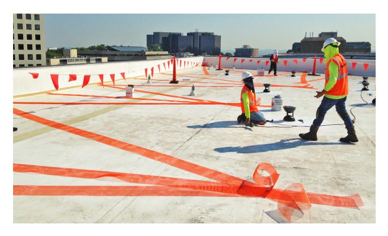
In total, 36 V2T vents were used - isolation vents to secure the existing roof and new vents for the recovery membrane. Fully installed as of mid July 2017, the property is now properly outfitted to weather even highly variable wind conditions, and because of the rapid installation, disruption to the downtown environment was minimized.
