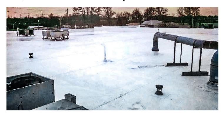
In 2016 there was a fire at the building next door and the Gilbreth roof suffered hundreds of burn holes. The V2T system still kept the roof in place even though the system was no longer sealed. While unfortunately the client had a massive roof repair issue the V2T system did its job and kept the roof in place even in winds.
