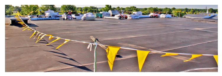
Insulation was 1½ inches of isocyanurate sprinkle mopped in place with an .045 EPDM membrane. A section of the south wall roof of the building had suffered delamination, and was currently mechanically attached. Clearly, an entire re-roof was in order to restore full usable function to the school.
