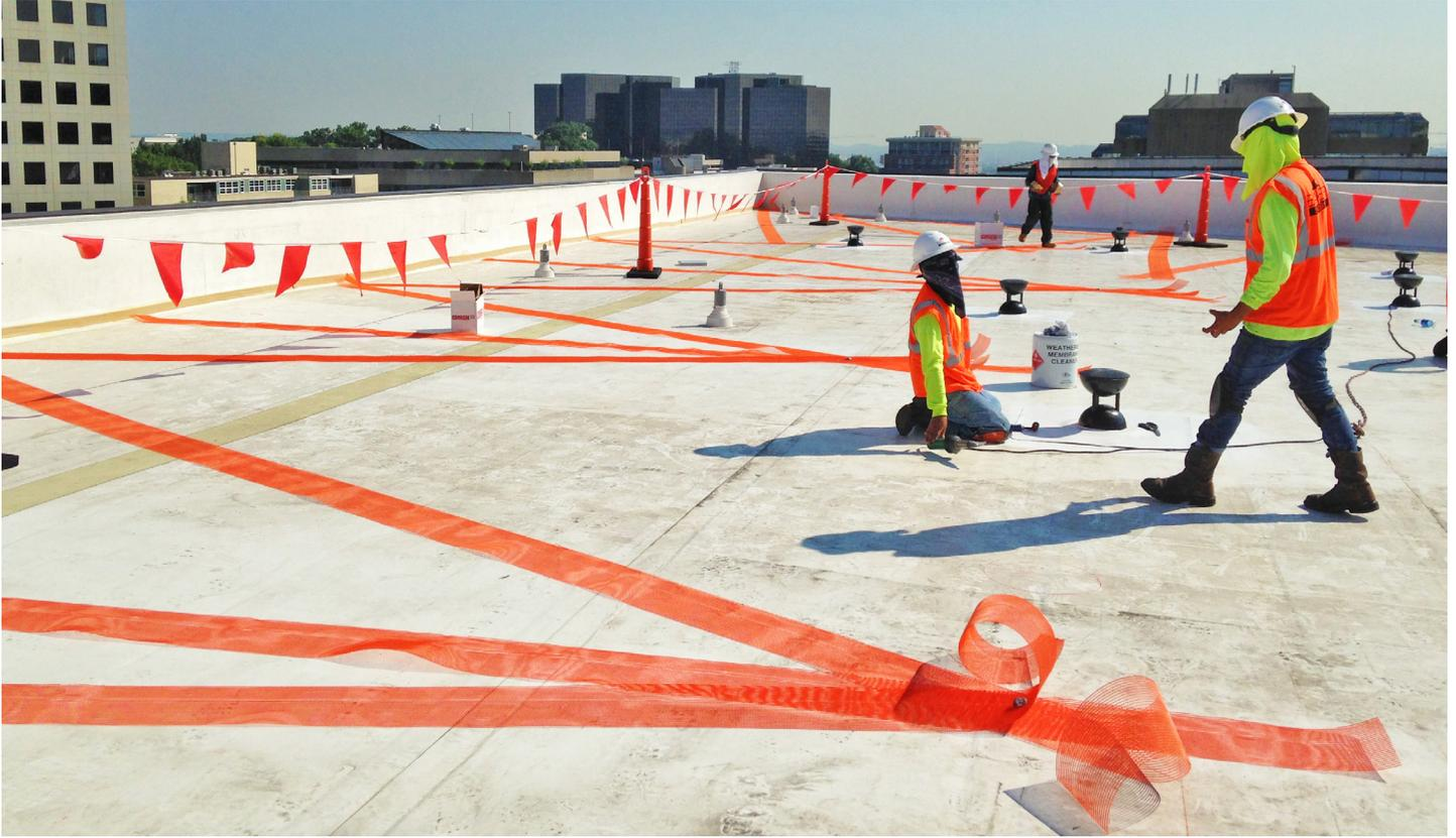
In total, 36 V2T vents were used - isolation vents to secure the existing roof and new vents for the recovery membrane. Fully installed as of mid July 2017, the property is now properly outfitted to weather even highly variable wind conditions, and because of the rapid installation, disruption to the downtown environment was minimized.
